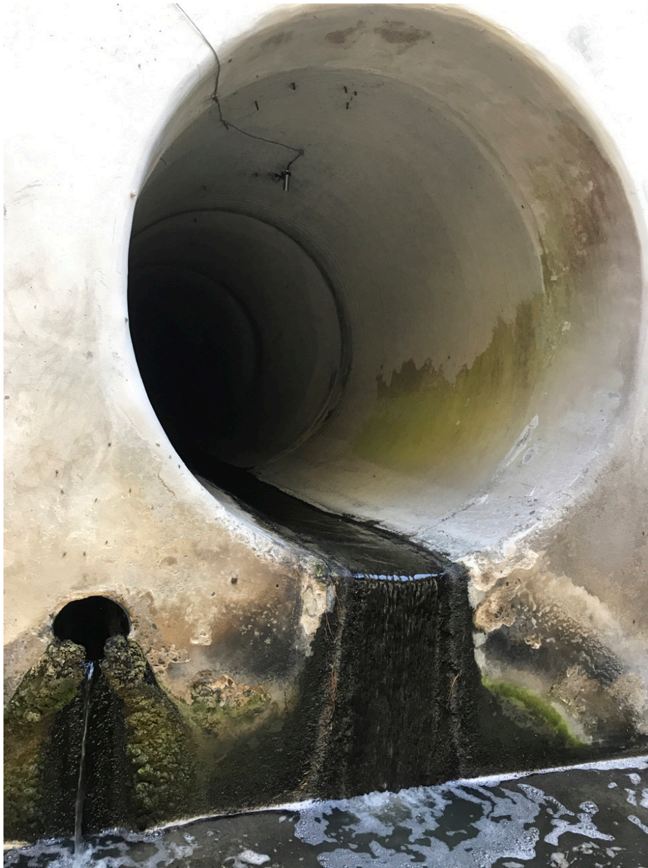
Figure 25. Inspection Photo of Outfall J03-9221-1
